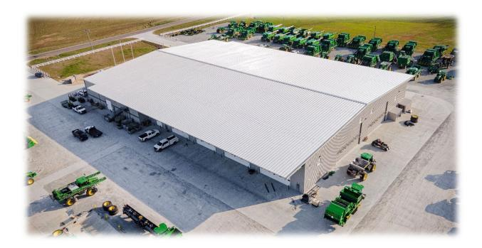
Kirby's Standing Seam 360 roof system in galvalume plus, as well as the R-Panel wall panels in fox gray were utilized. The lean-to ceiling is fully lined and complete with Kirby's Loc Seam roof panels in slate gray.
